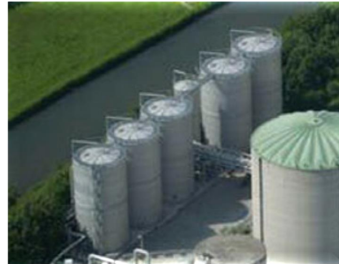
WABAG UASB (Upflow Anaerobic Sludge Blanket)
